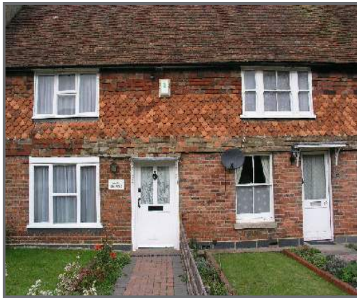
A typical village cottage with attractive half tiling and a pleasant door, but with not entirely suitable replacement window frames. The cottage on the right is the reverse, with slightly better windows, but an unsuitable door.
