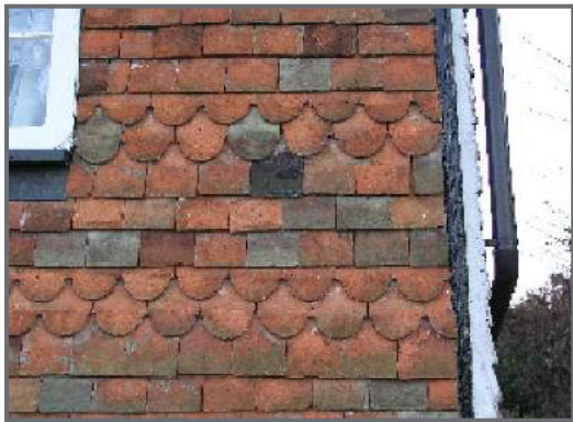
Half tiling with fish scale tiles - a paterend mix
