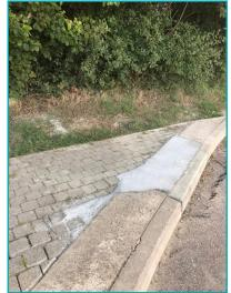
The footpath was repaired between Lodge Close and Cuckoo Park after the concrete broke down and bricks came loose
