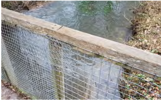
Bridge at Singleton Lake repaired
