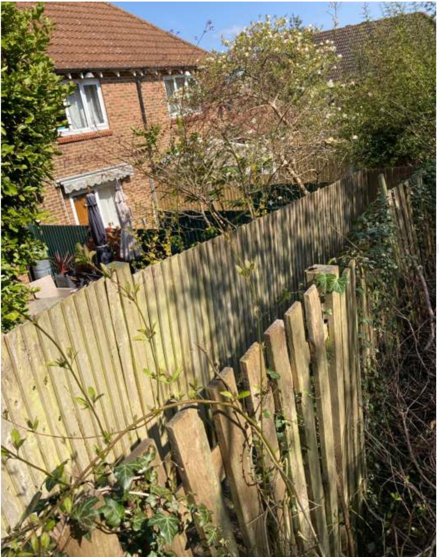
Fig.7 Walkway at rear of properties
