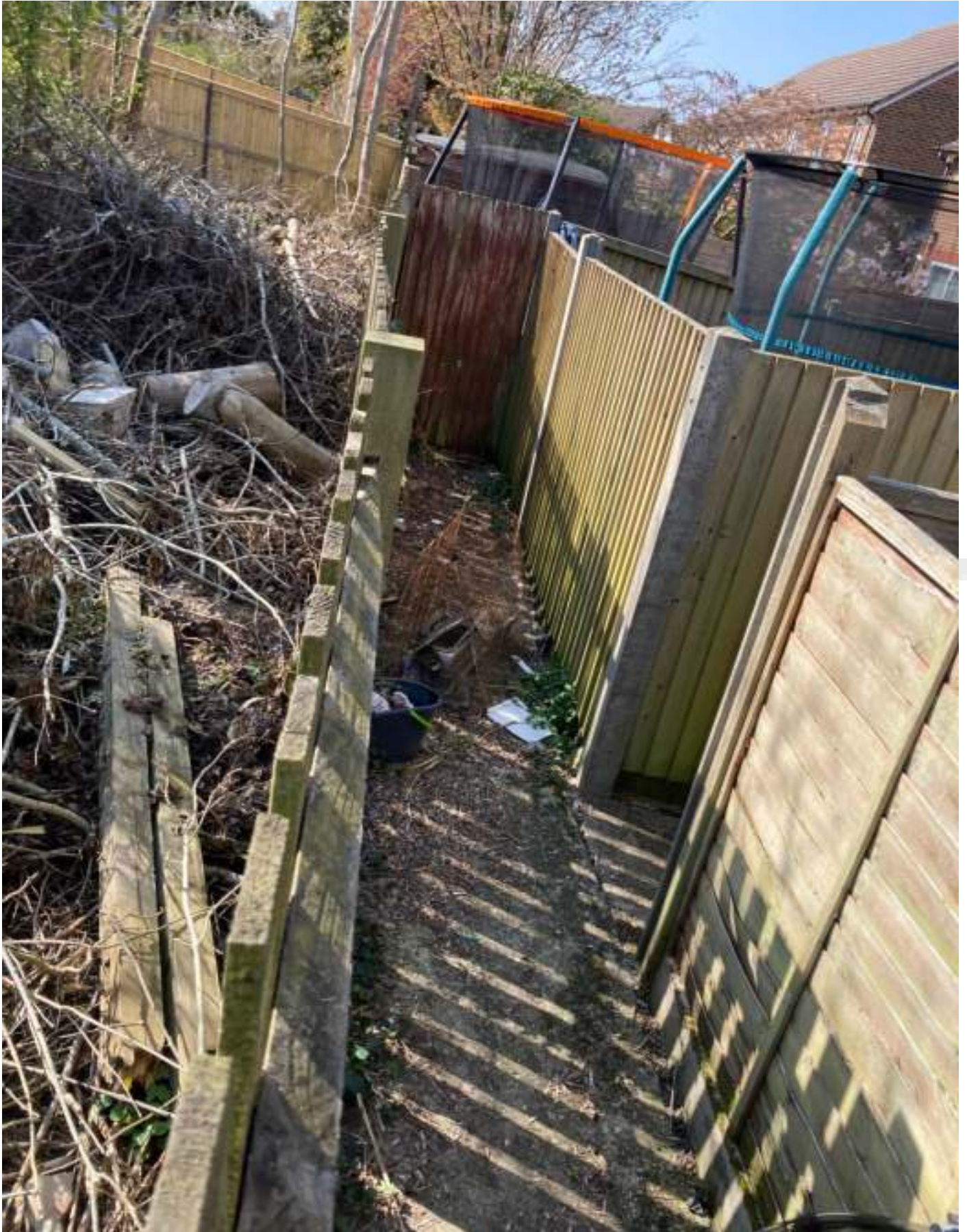
Fig.6 Walkway at rear of properties
