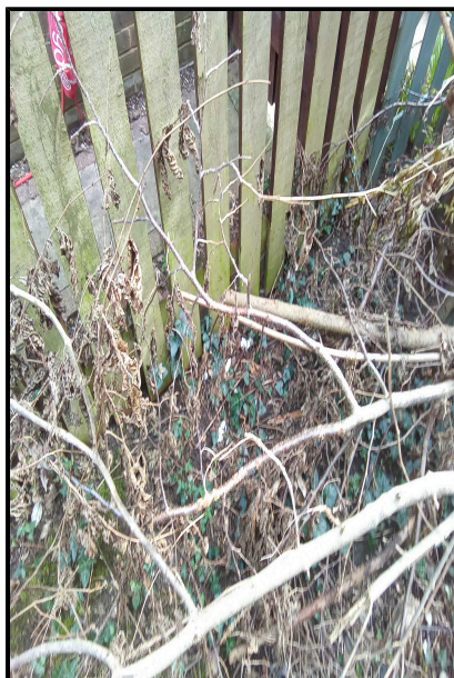
Inspection carried out along the fenceline of bradbridge green carried out.
